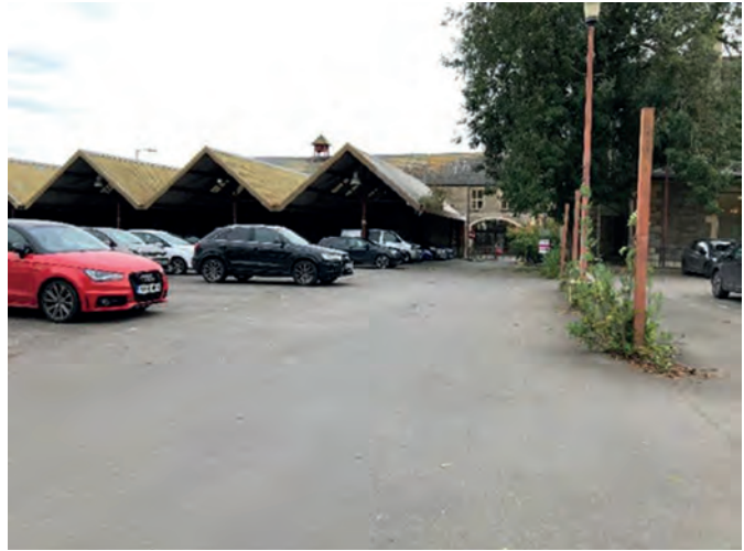
No demarcated pedestrian routes makes for exclusionary design, Bath Road Car Park
