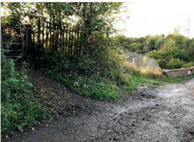
No waymarking for the public footpath (left), despite this being the most direct walking route to the town centre from this location on Cocklebury Lane
