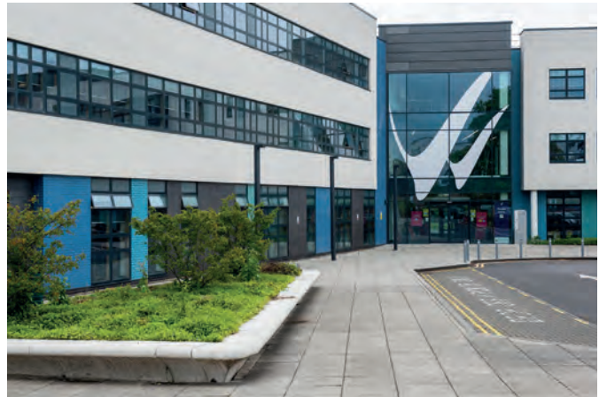
Wiltshire College is the only BREEAM 'Excellent' building in Chippenham
