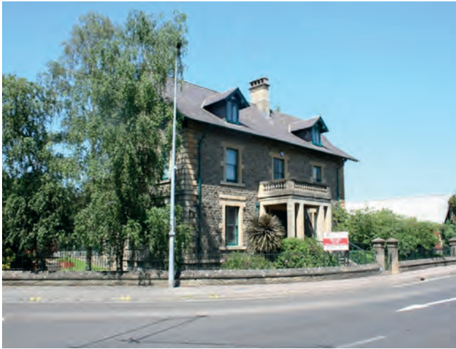
The Grade II Listed Bank House fronts on to Bath Road and sits in isolation on the site
